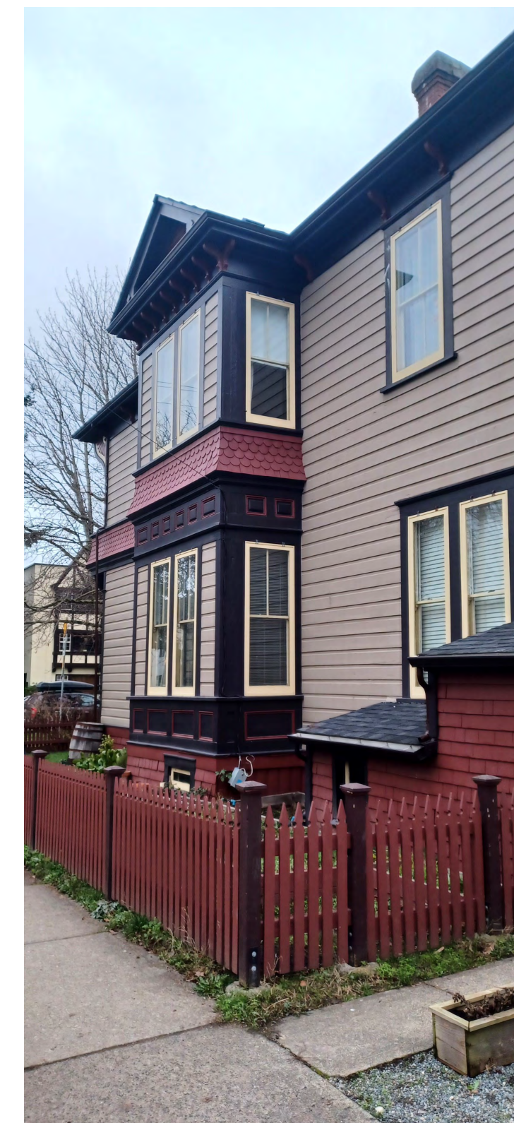
Douglas Fir heritage window installed within the sunken courtyard will match existing colours
