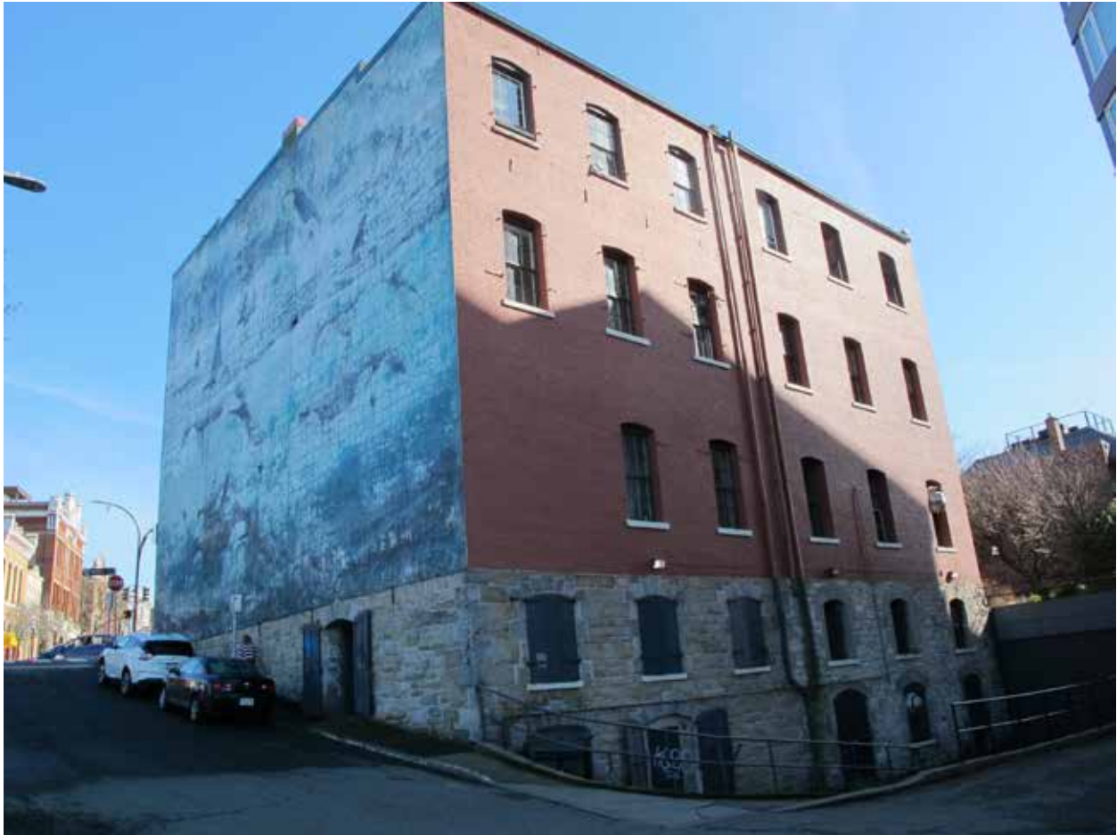
Rear (right) and north (left) elevations of the Yates Block showing painted brick on rear elevation and painted mural installation on north elevation
