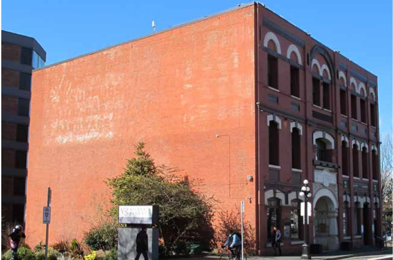
South elevation (left) of the Yates Block with ghost lettering of past painted signage.
