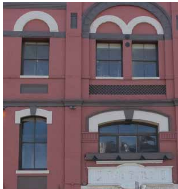
Below: Windows of front elevation including 2-over-2, hung, segmental arch wood windows; 2-over-2, hung, wood windows; and triple assembly wood window with multi-lite segmental arch transom.
