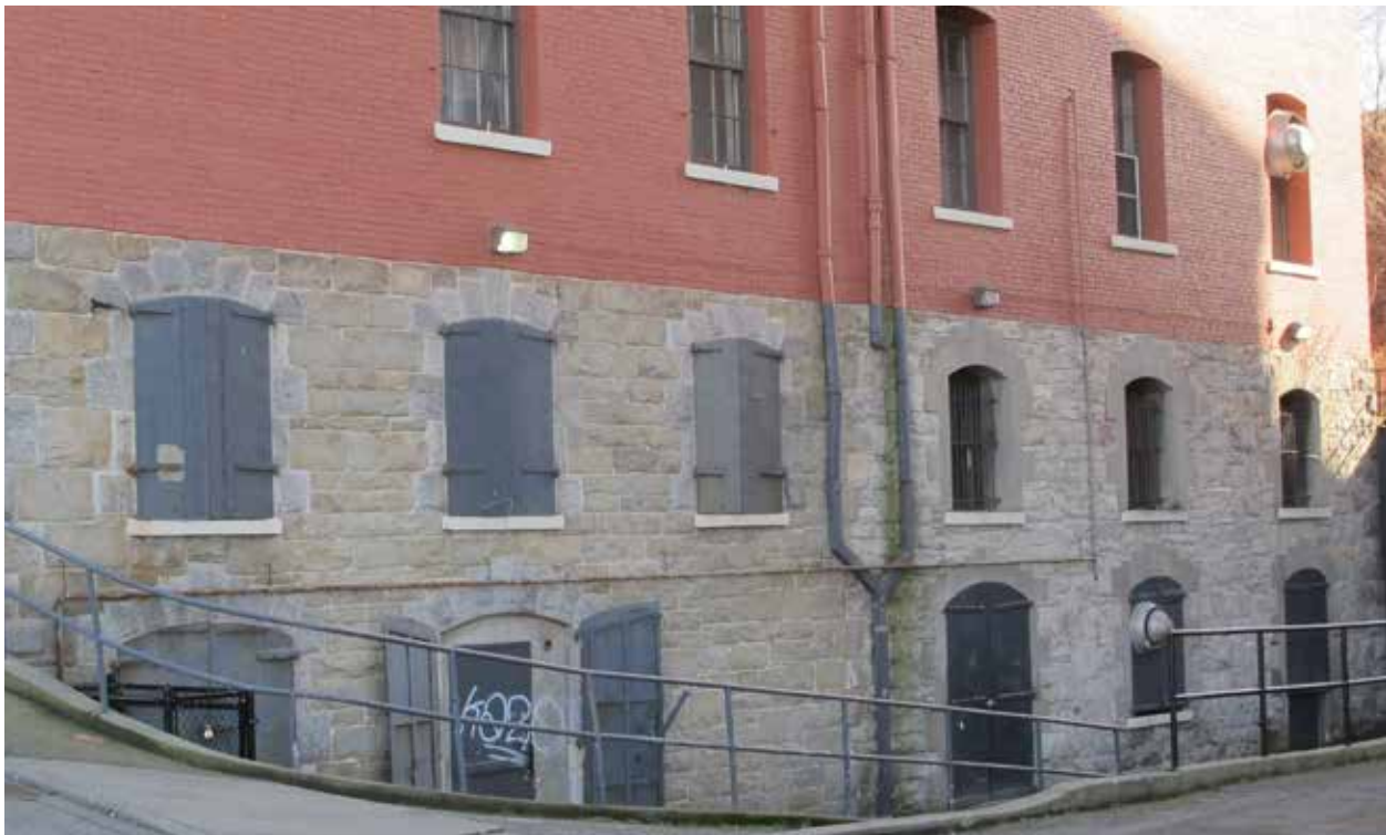
Rear elevation of the Yates Block with four doors providing access to the building's lowest level.
