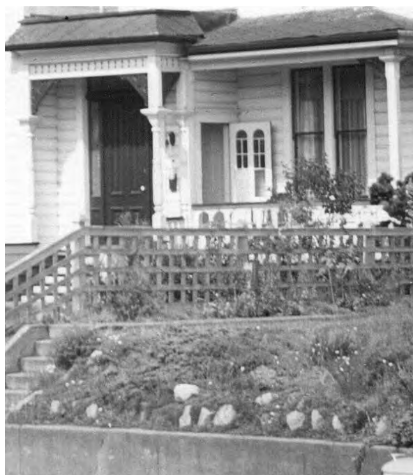
Left Top: Extant front door with sidelights. Note original multi-lite sidelights and door knob have been replaced.
