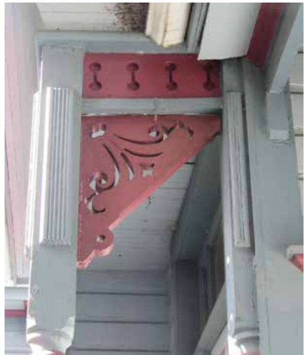
Above: Front entryway porch with flat hipped roof, low closed balustrade, lathe-turned fluted posts, and decorative frieze and brackets. Original gabled cap on top of balustrade is replaced. Below: Close up of original decorative frieze and brackets and top of lathe-turned post.
