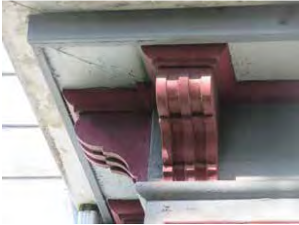
Above: Original scroll cut brackets of bay window roof.
