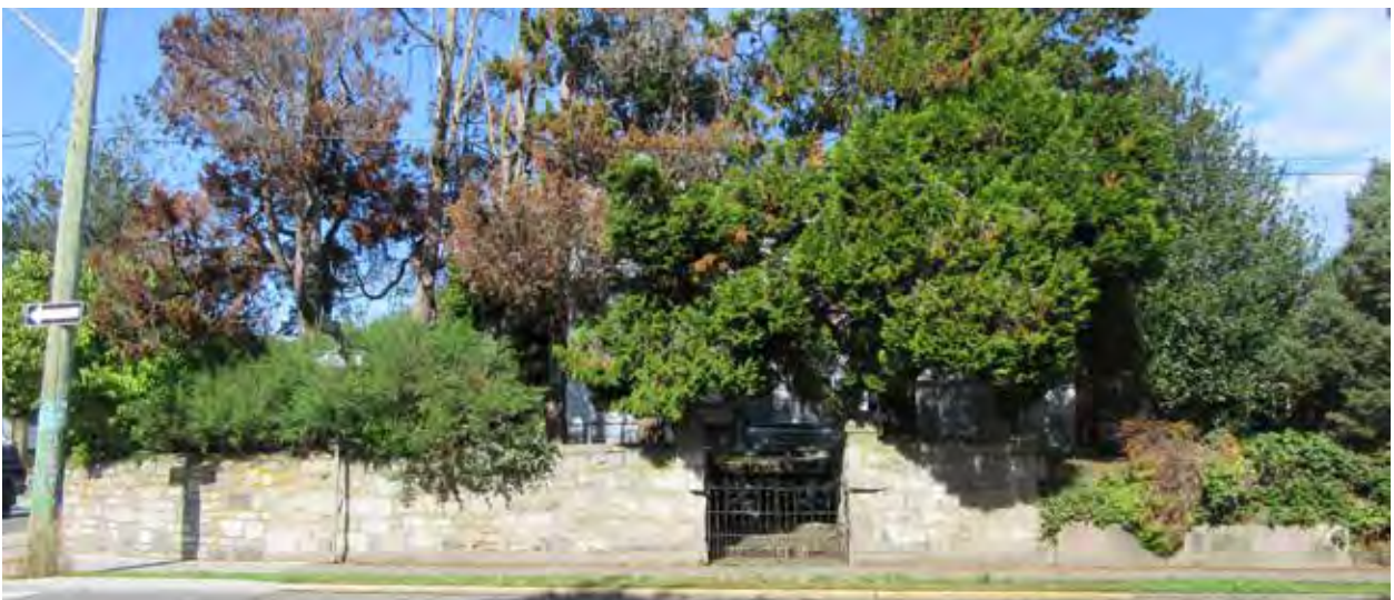
Top: Original curved granite retaining wall at Pandora Avenue and Fernwood Road property lines. Middle: Granite retaining wall and square gate posts at existing vehicle entry off Fernwood Road. Bottom Right: Pedestrian entry with wrought iron gates off Pandora Avenue.
