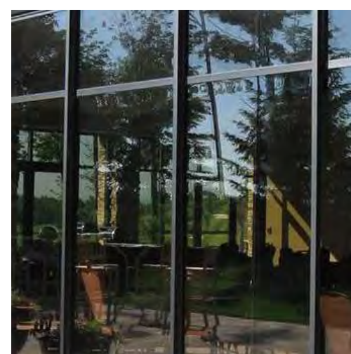
CW CURTAIN WALL BLACK MULLIONS
