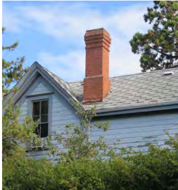
Above: Original internal red brick chimney with corbelled cap.
