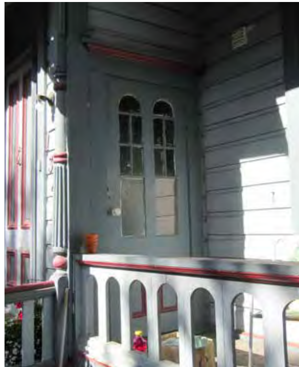
Above: Original wood door to front porch with multi-lite glass panels.
