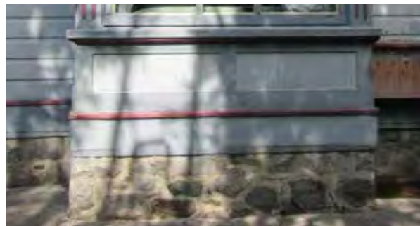
Above: Vertical tongue-and groove spandrel panels below bay window.
