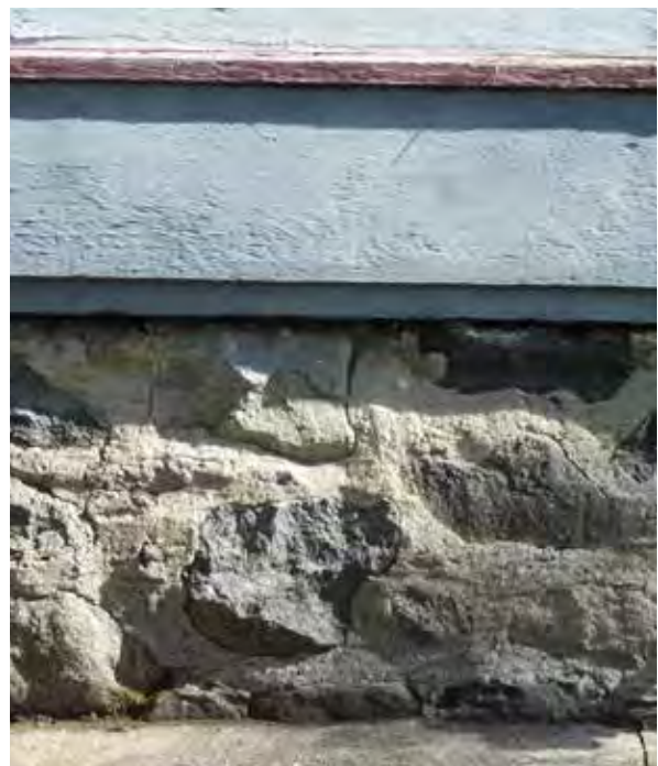
Above: Intact original field stone foundation.
