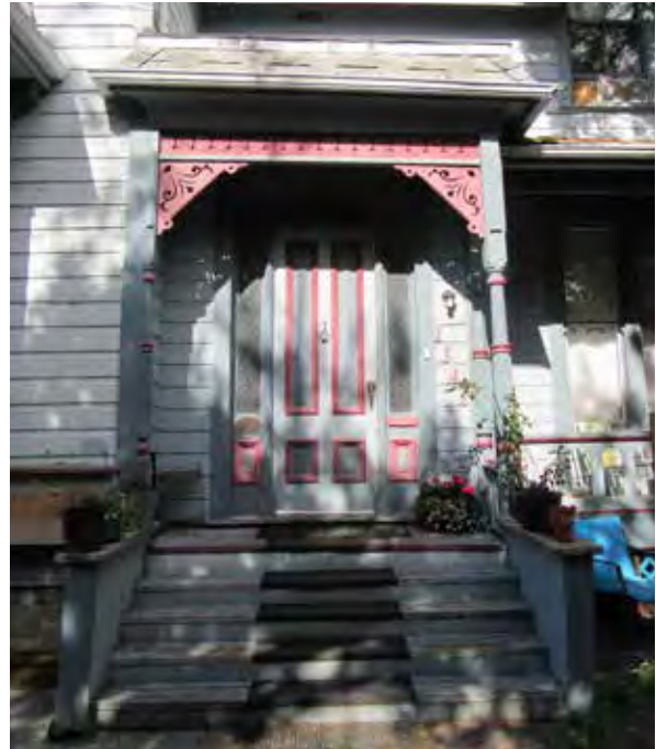
Above: Front entryway porch with flat hipped roof, low closed balustrade, lathe-turned fluted posts, and decorative frieze and brackets. Original gabled cap on top of balustrade is replaced. Below: Close up of original decorative frieze and brackets and top of lathe-turned post.
