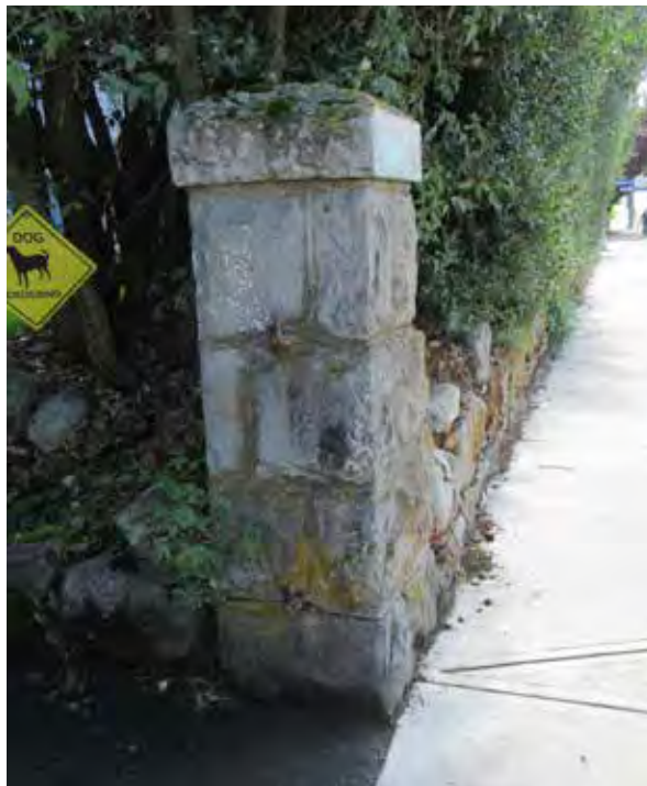
Above: Square granite gate post at vehicle entry with iron bolts indicating a gate existed at this entry at one time.
