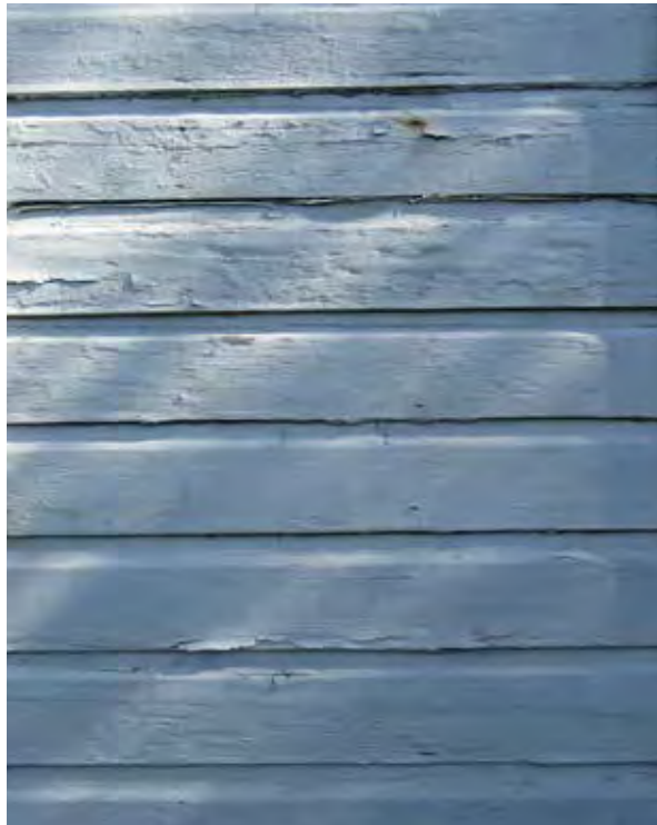
Above: Vertical tongue-and groove spandrel panels below bay window.
