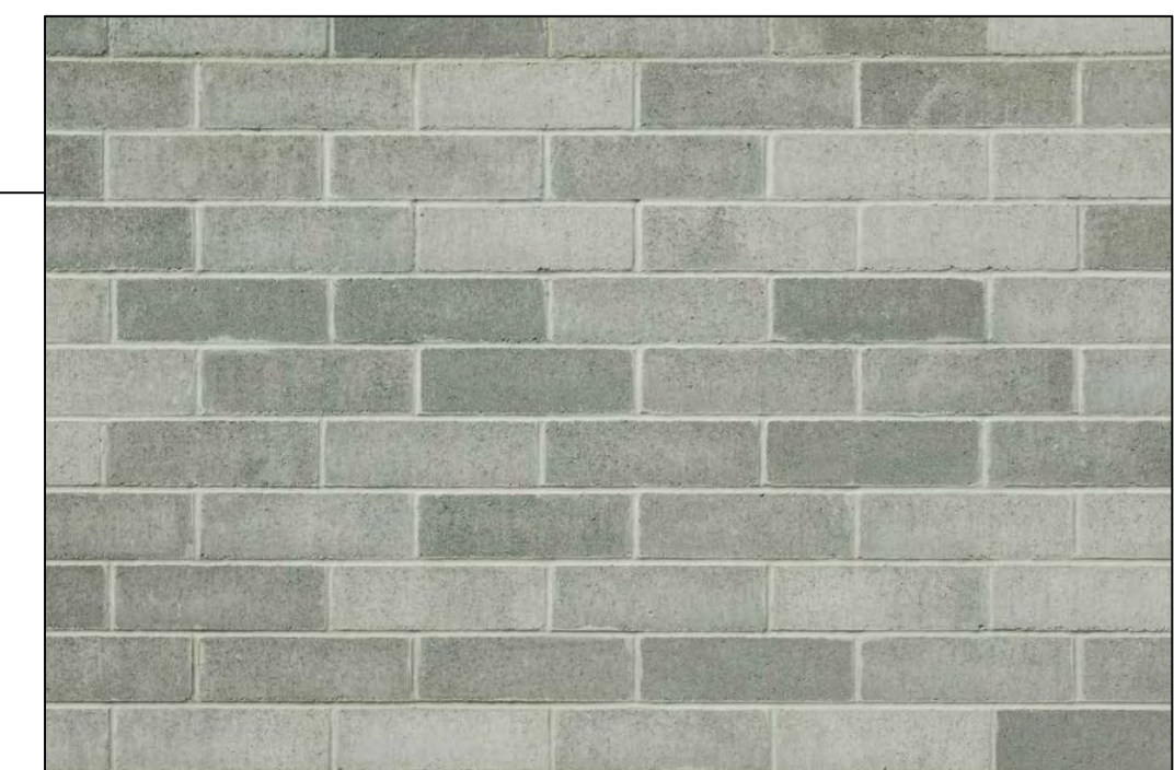
Smooth face masonry cladding
