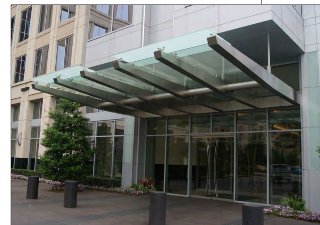
Steel and glass canopy
