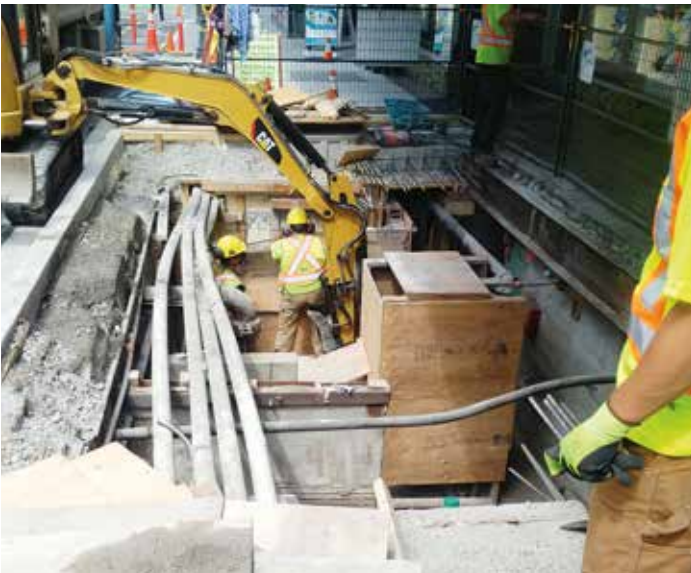
City carpenters working on Fort Street.
