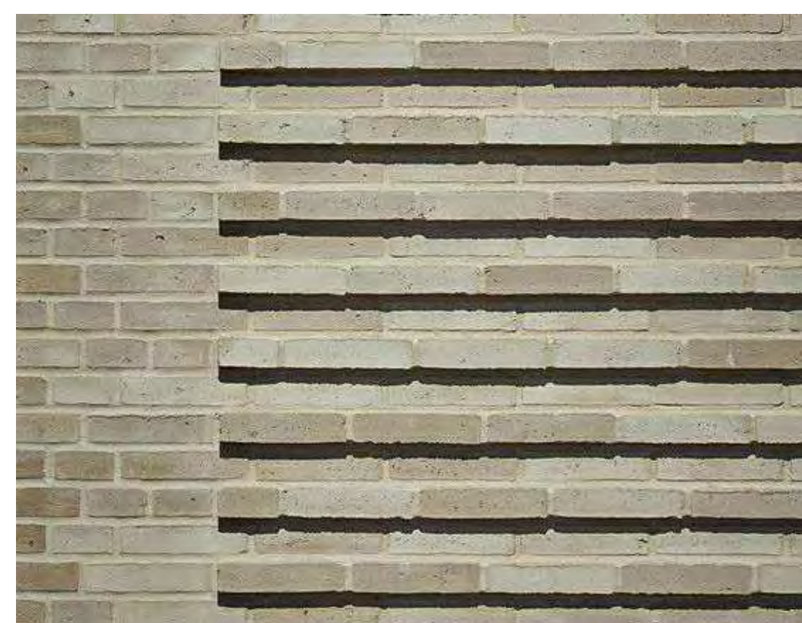
HORIZONTAL BRICK REVEAL DETAILING
