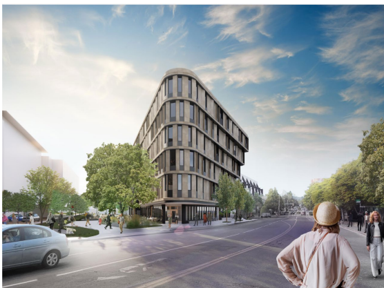
Figure 1: Street level view from Richmond Road looking north
