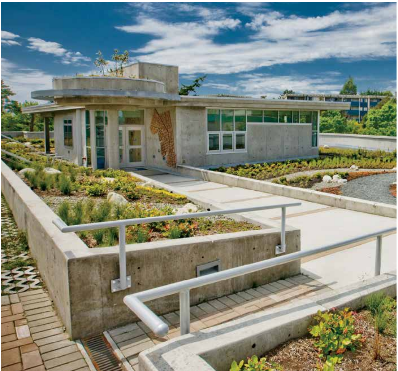
Burnside Gorge Community Centre green roof.
