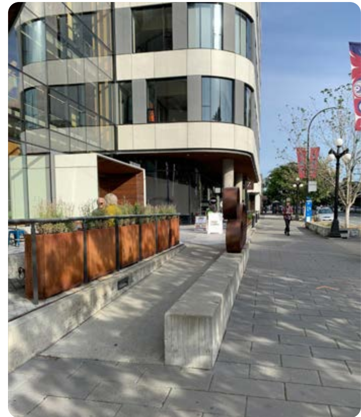
Example of a highly visible access ramp integrated into overall building design.
