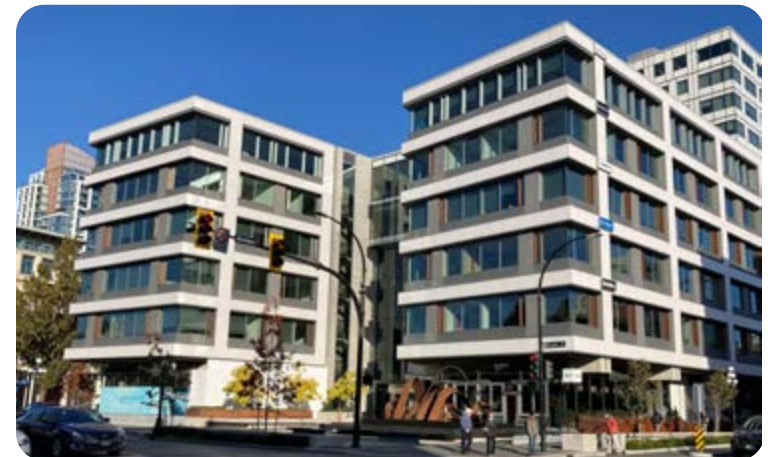
Example of incorporating a vertical break in the building facade associated with a lobby entryway.
