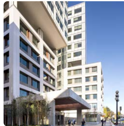
Example of a tall commercial/office building incorporating a combination of upper storey recesses, projections and stepbacks to articulate building mass.
