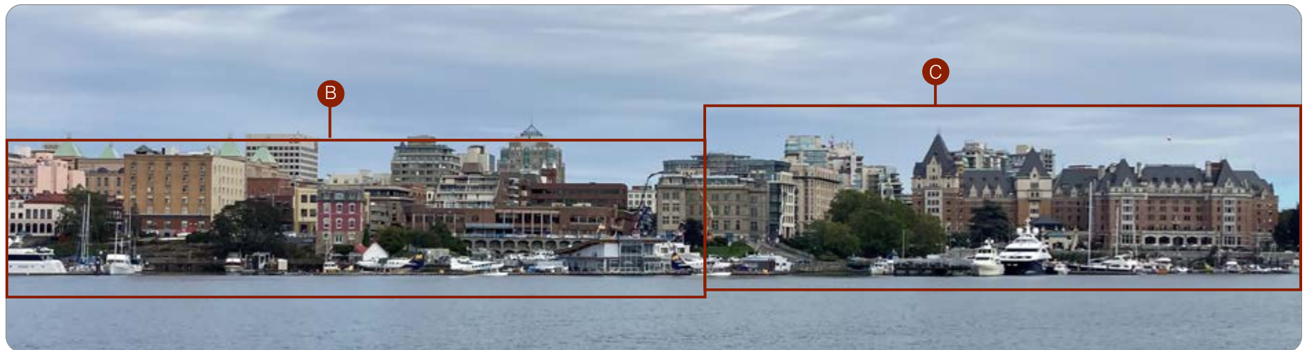
Laurel Point looking Southeast
