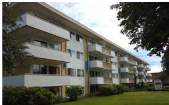
Rental apartment buildings
