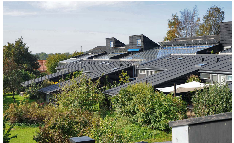
Skylights and roof monitors enable these dual-aspect family-friendly townhomes that are otherwise flanking a central community atrium. [Vandkunsten - Savvaerket Cohousing; Image credit: Vandkunsten]
