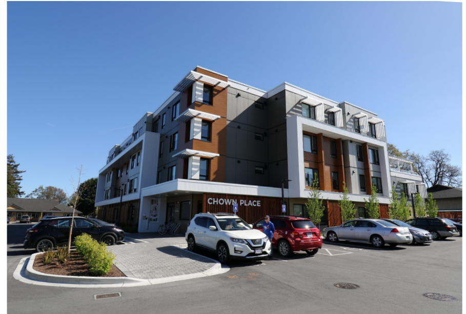
Three-bedroom homes of 98 sq. m. (1,054 sq. ft.) floor areas can be found at Chown Place, a family-friendly and affordable apartment building in Victoria. [Image credit: City Staff]
