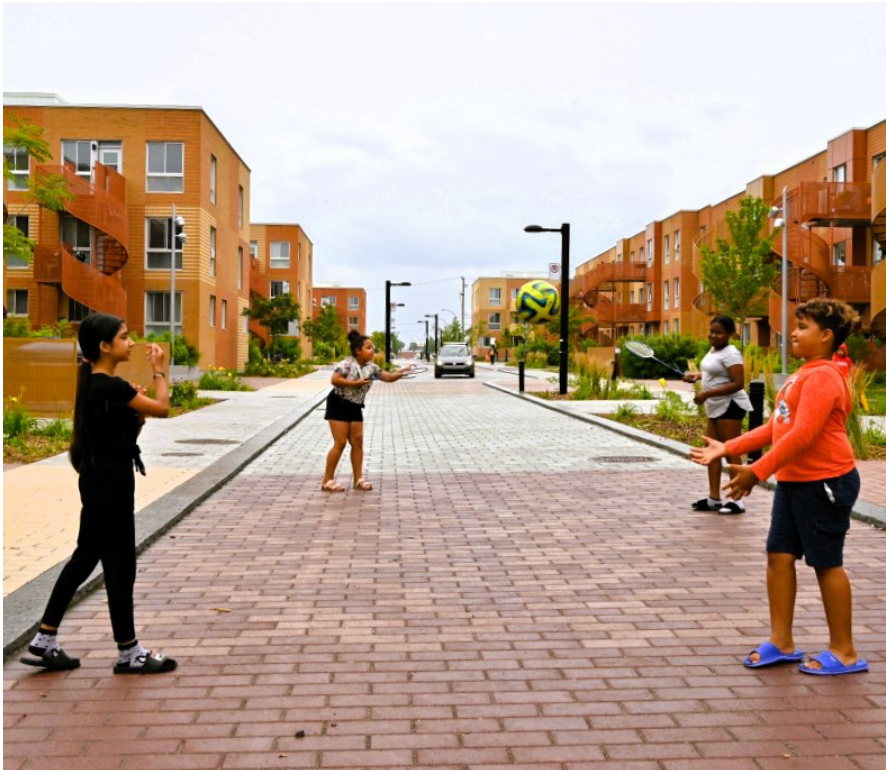
The built form and shared-traffic laneway of this affordable Montreal development encourage social interaction among residents. [Saia Barbarese Topouzanov architectes and Vlan Paysages – Habitations Saint-Michel-Nord; Image credit: James Brittain]
