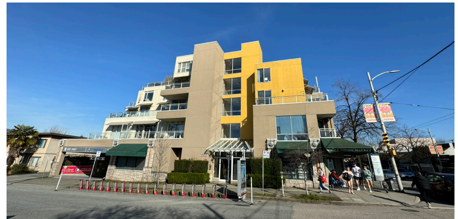
Daylight access to elevator lobbies and corridors can be seen from the outside of this family-friendly, mixed-use development in Vancouver. [Hotson Bakker Architects - 1978 Vine Street (Capers Building)]; Image credit: City Staff]
