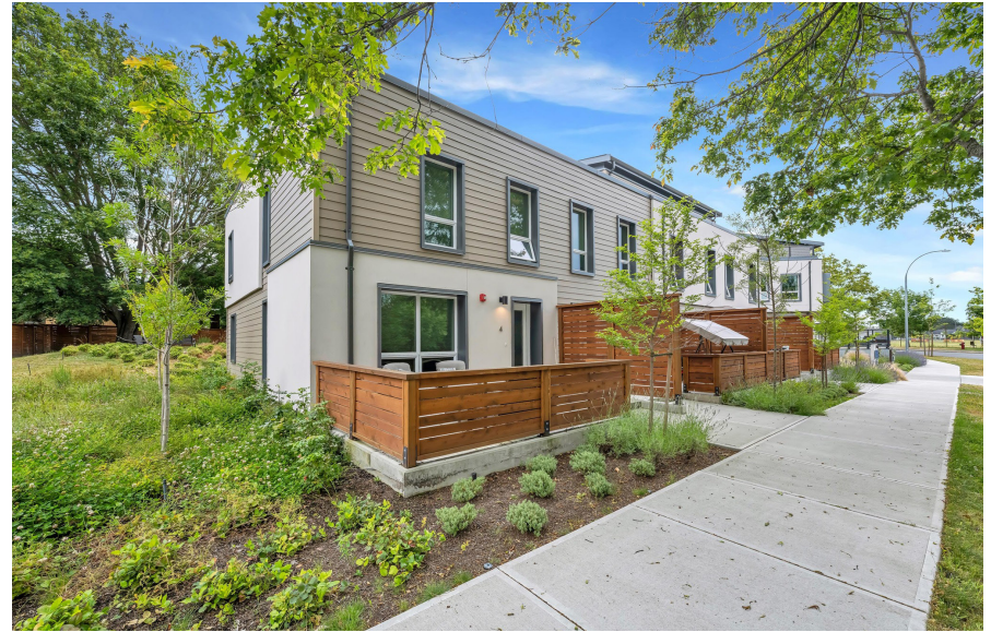
Family-friendly Saanich townhomes include private patios, privacy fences and strategically located deciduous trees for seasonal shading. [HCMA Architecture + Design - Townley Place Affordable Housing; Image credit: H&R Exterior Finish]
