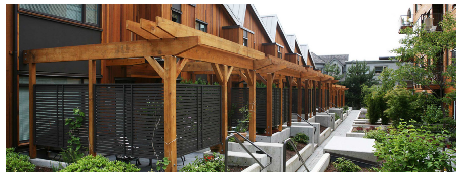
Raised private patios with privacy screens and solar shading improve the family-friendly livability of these Saanich townhomes. [DAU Studio - Richmond Gate Housing; Image credit: DAU Studio]
