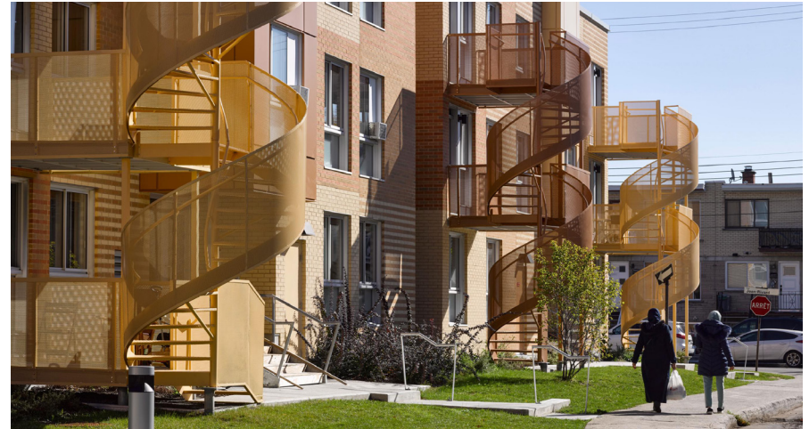
A Montreal affordable housing development offers direct means of access for each residence. [Saia Barbarese Topouzanov Architectes and Vlan Paysages – Habitations Saint-Michel-Nord; Image credit: James Brittain]
