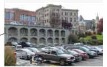
Parking Lot and Retaining Wall
