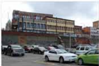
Parking Lot and Historic Retaining Wall
