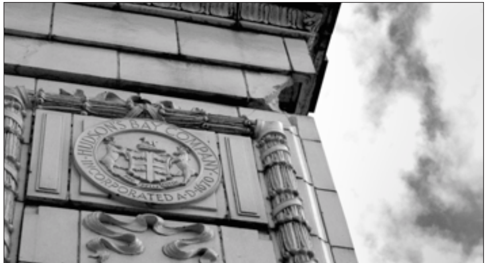
figure 5 — existing Bay building façade
