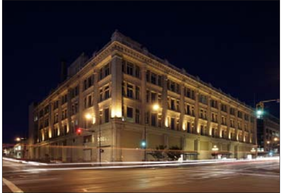
figure 4 — existing Bay building at the corner of Douglas and Fisgard
