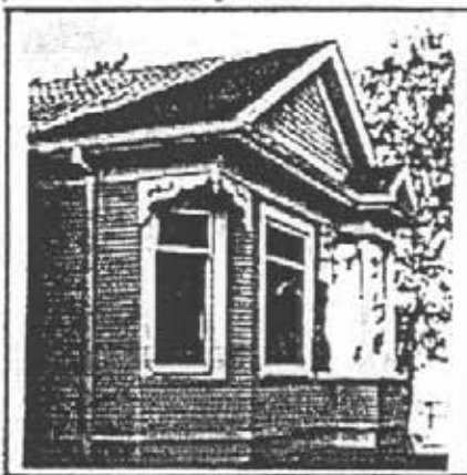
Projecting porch, chamfered corner, pronounced building base.
