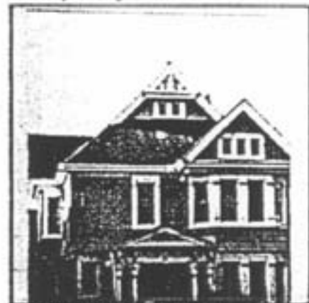
Combinations of roof pitches.
