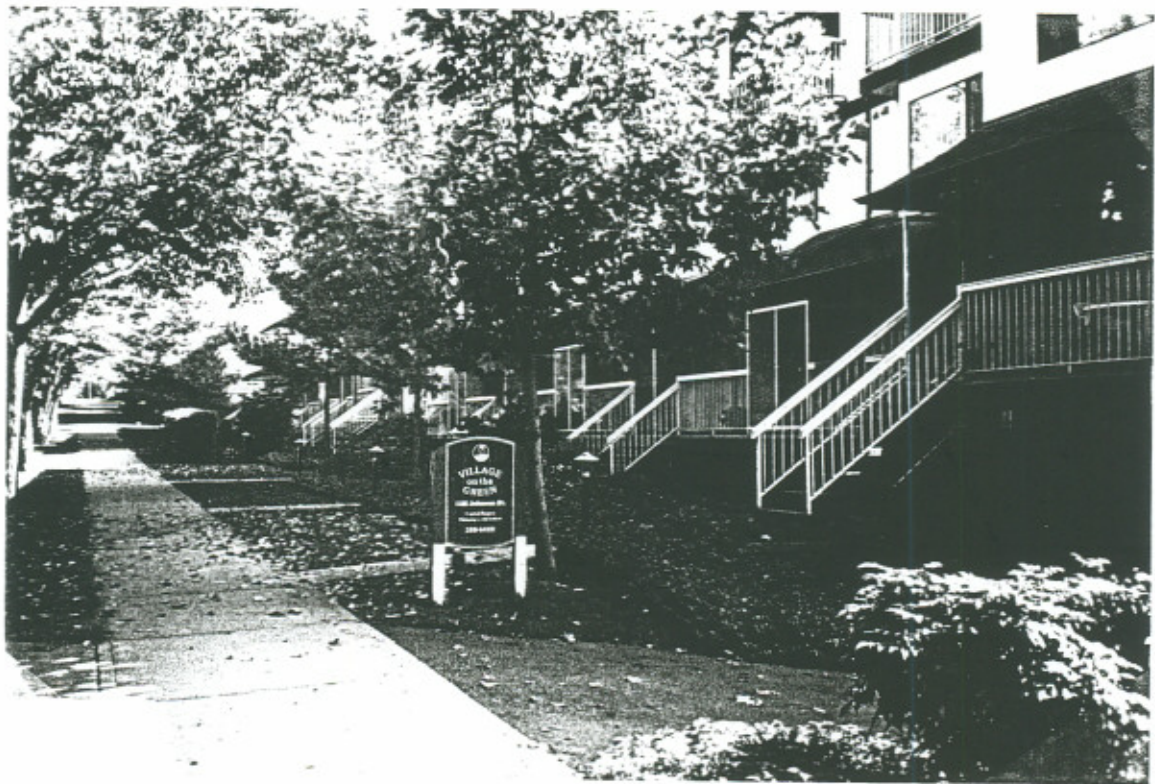
Village on the Green – stacked townhouses / Victoria Number of units = 38 Density = 32 units per acre
