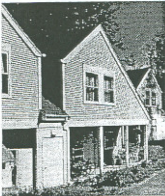
Figure 9 - Sawtooth roof and wood siding
