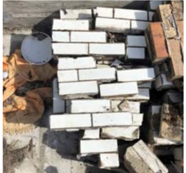
Representative condition of the bricks
