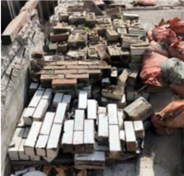
Stockpile of the salvaged glazed white bricks
