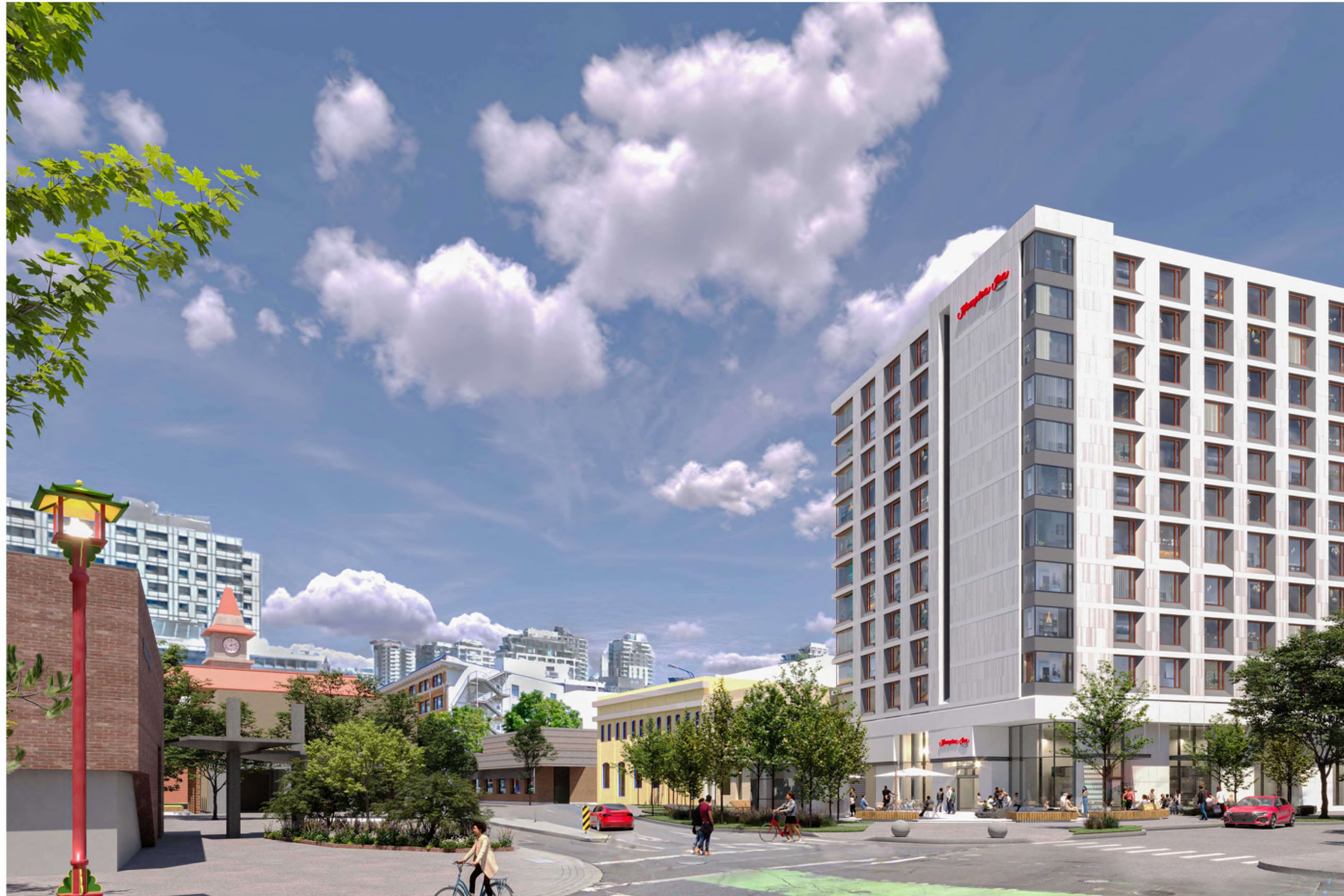
1. VIEW FROM ACROSS PANDORA AVE & GOVERNMENT STREET
