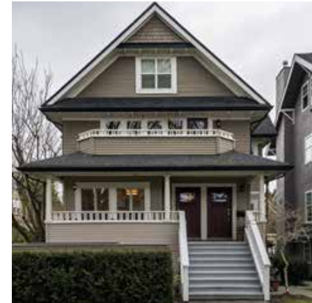
Figure 27: Example of heritage house converted to a duplex
