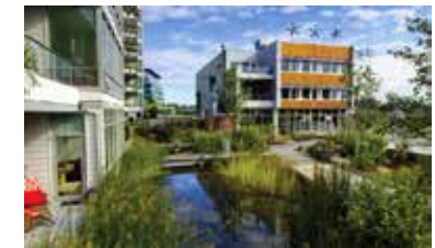
2008: First residents move into Dockside Green, a green mixed use development on a former industrial site.
